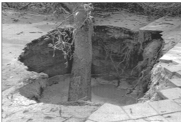
Figure 3. The sink-hole which engulfed part of the Świerczewski Street and a pavement with a tree
