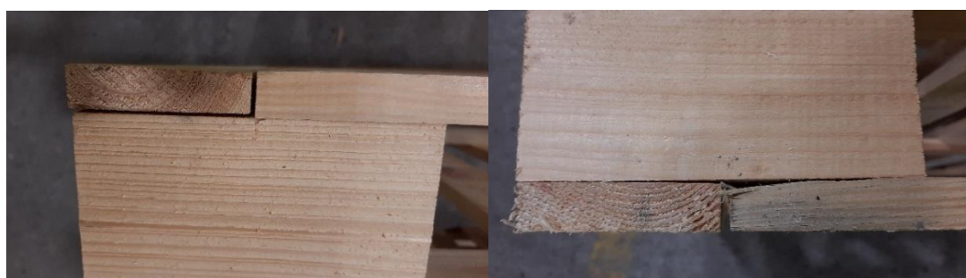
Figure 4. Construction joints Source: own elaboration.
